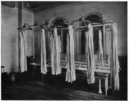
Courtesy Utica Drop Forge and Tool Co. Bathroom for Employes Finished in Glazed Brick.
